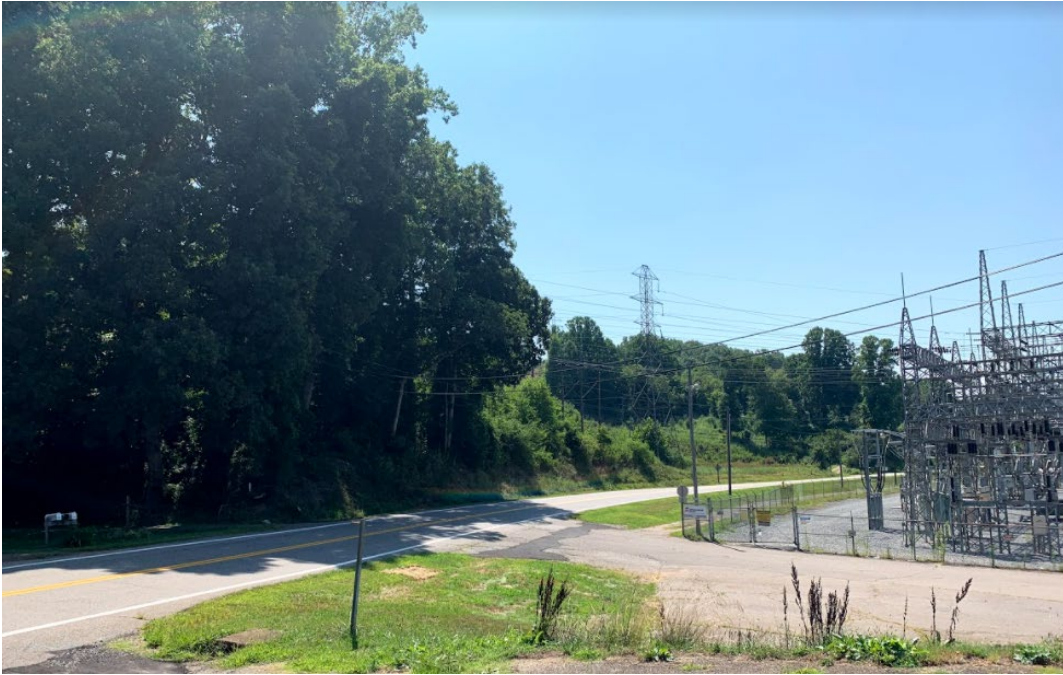
Photo 1. Appalachian Drive and Fieldale Substation
